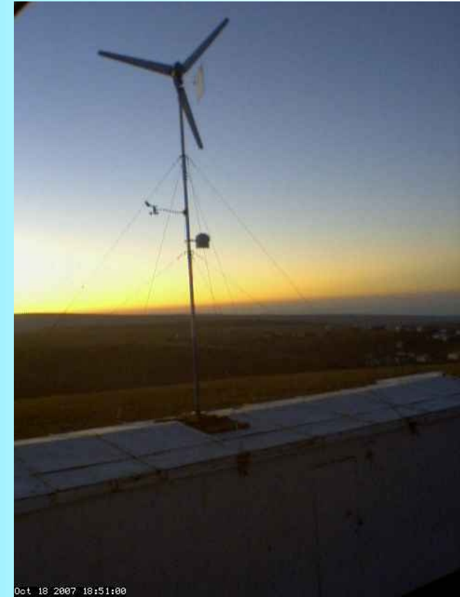
October. Evening. Yard-space control camera
